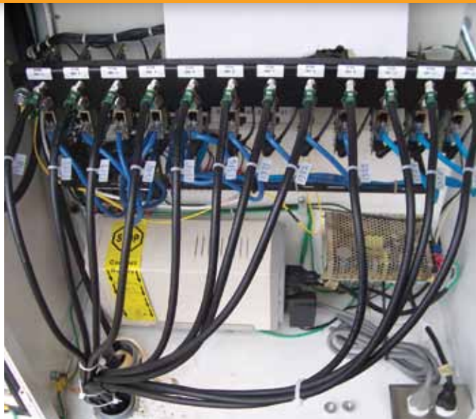
Figure 3: Connexion IDF Cabinet
